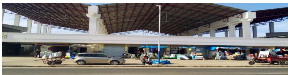
Plate 2: Iringa Urban District Newly Constructed Market at Mlandege Ward
